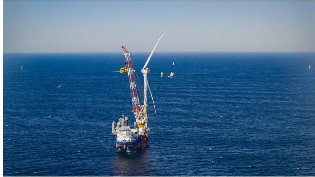
First (11 MW) Turbine Installed at South Fork Wind, November 2023
