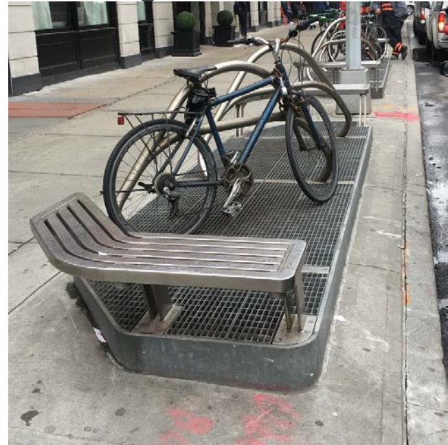
Fig 18.10- Subway Air Vent Flood Protection
